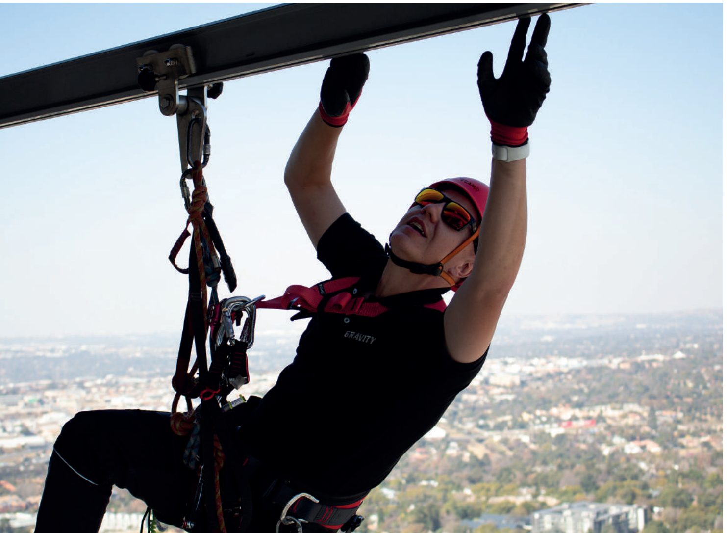
Martyn Cilliers doing maintenance operations on the Leonardo building, using C.A.M.P. gear and the Gravity Securail. Martyn Cilliers realiza el mantenimiento del edificio Leonardo, utilizando equipos C.A.M.P. combinados con Gravity Securail. Sandton, Johannesburg, South Africa (courtesy of Gravity Gear Pty Ltd, ph. Ethan de Witt).
