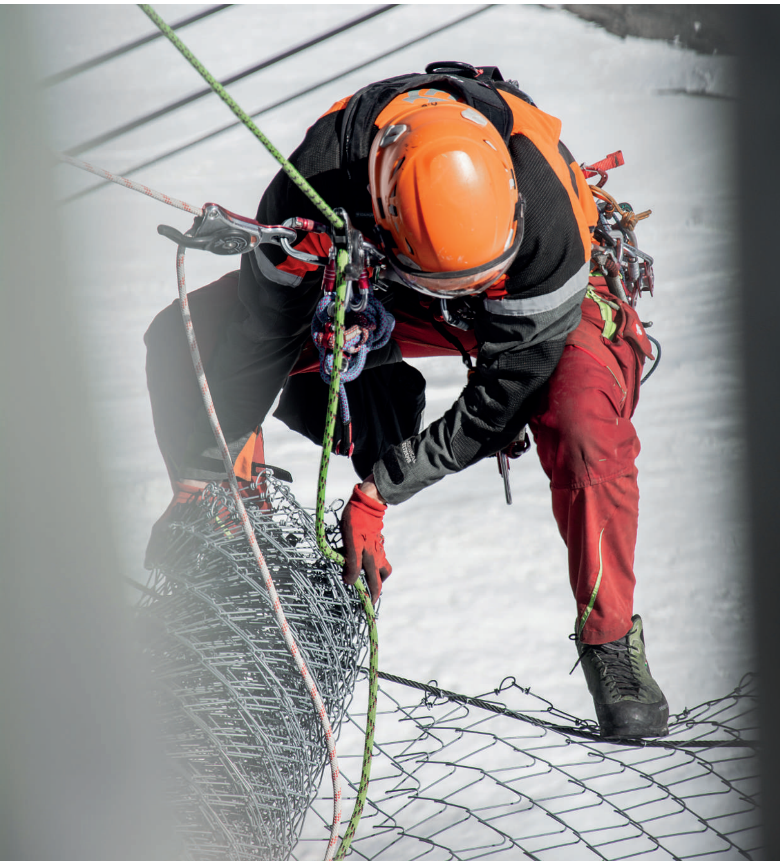
Installation of anchor points and safety nets for the reconstruction of the famous "La Botta" restaurant at Glacier 3000. Instalación de anclajes y redes para la reconstrucción del famoso restaurante «La Botta» en Glacier 3000. Les Diablerets, Switzerland (courtesy of Corde-Access SA, riggers Andrea Giazzi & Julien Guisolan, ph. Ari Cretton).
